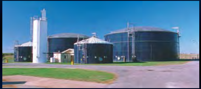
▲ Sludge stabilization and sludge storage facility.
