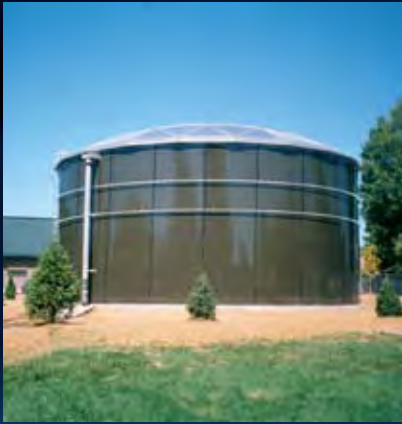
Ground Storage Tank
